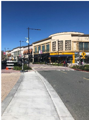
Broadway Plaza Phase I, Walnut Creek
